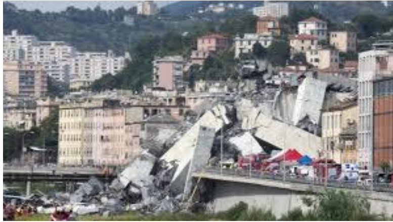
Figure 20 – Collapse of Genoa bridge in 2018
